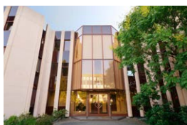
Pully (VD) Avenue Charles-Ferdinand Ramuz 43
